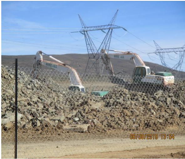
Photo: Breaking of rock at section D.
