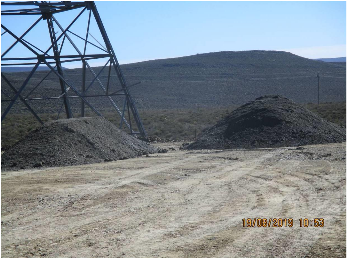
Photo: Import material (G6) to be used as final layer or wearing course.
