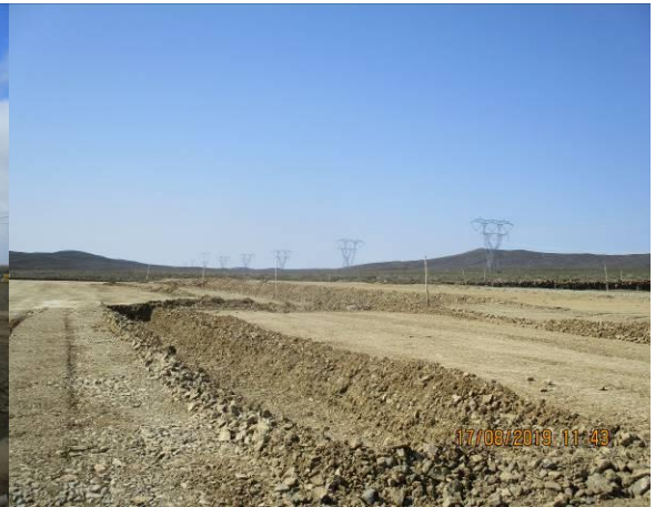
Photo: Preparing retaining wall foundation
