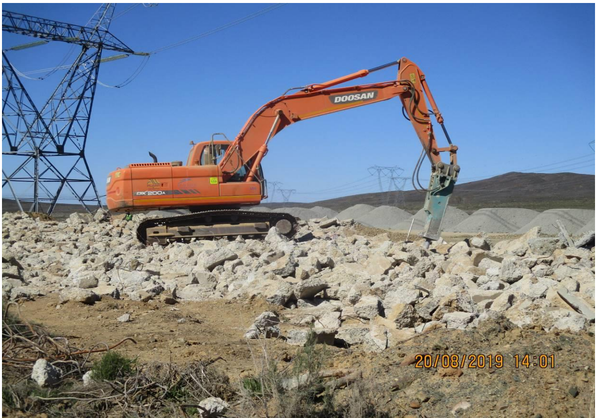
Photo: Breaking of concrete waste to be reused as backfilling material.
