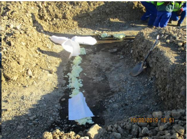
Photo: Hydraulic pipe burst from bomag roller. Photo: cleaning in progress.
