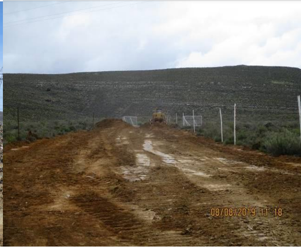
Photo: Construction of permanent access road
