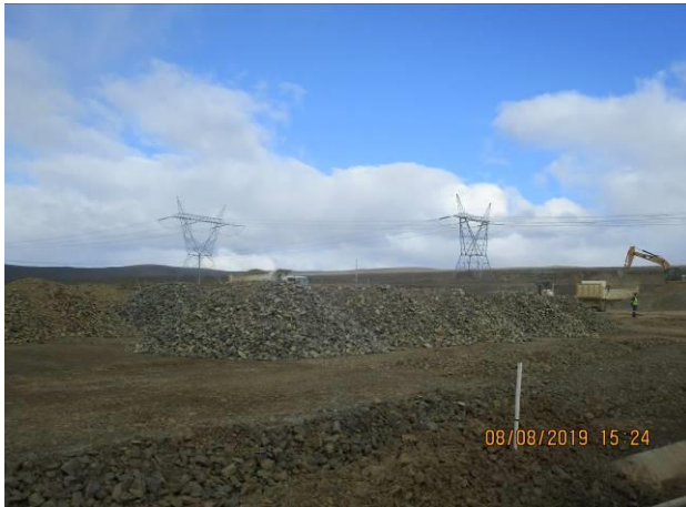
Photo: Layer works at section B (132kV terrace).
