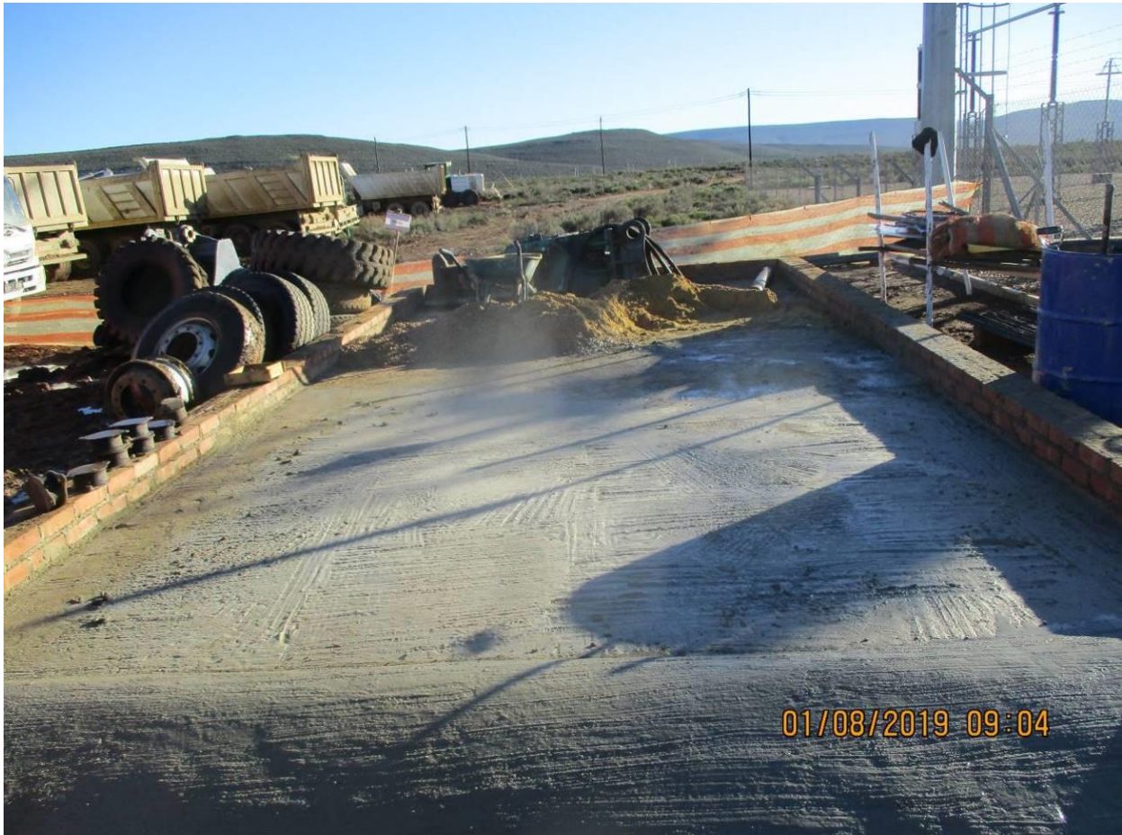
Photo: Vehicle servicing area.
